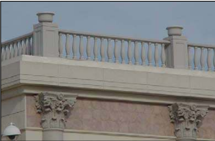
Balustrade as parapet wall • Architectural Fiberglass (GFRP)
