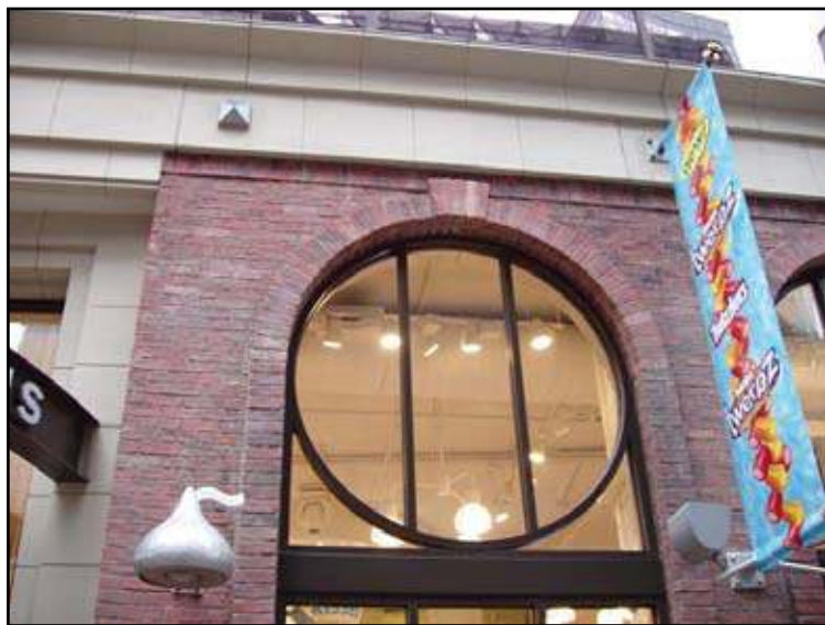
Architectural fiberglass brick panels, Hershey's Times Square, New York
