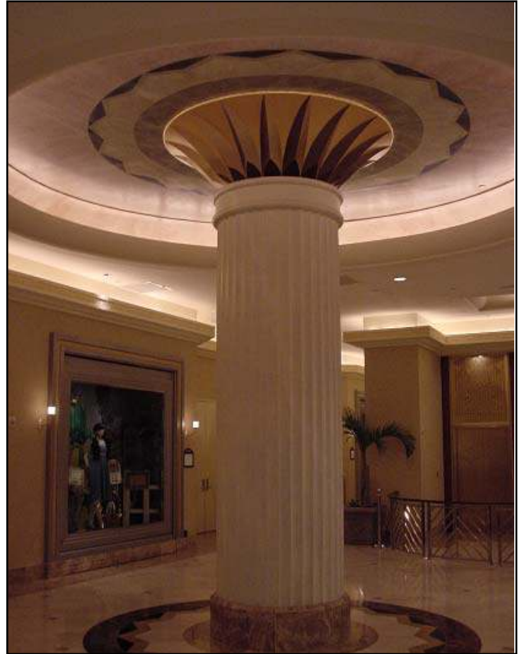
Column in architectural fiberglass with a GFRG capital and GFRG light cove.
