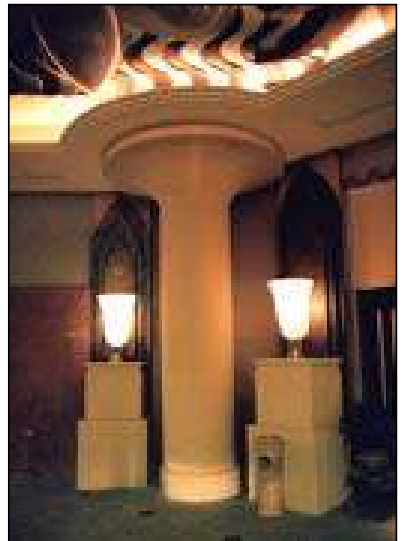
Column in architectural fiberglass with a GFRG capital and GFRG light cove.
