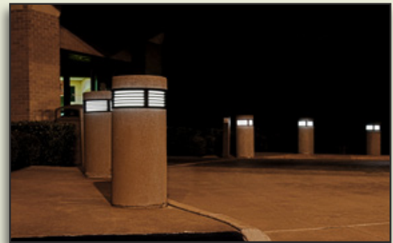
Illuminated Bollards, Hospital
