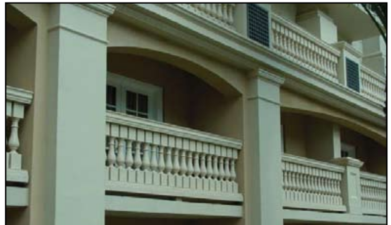
Balcony railing for a hotel and resort. This balustrade railing was delivered and installed in full sections. The ends have clips for attachment to the structure. This balustrade / railing meets all the code requirements for height, spacing and strength. Water drainage for the balustrade is accomplished with the raised bottom rail. Material is Stromberg architectural fiberglass.
