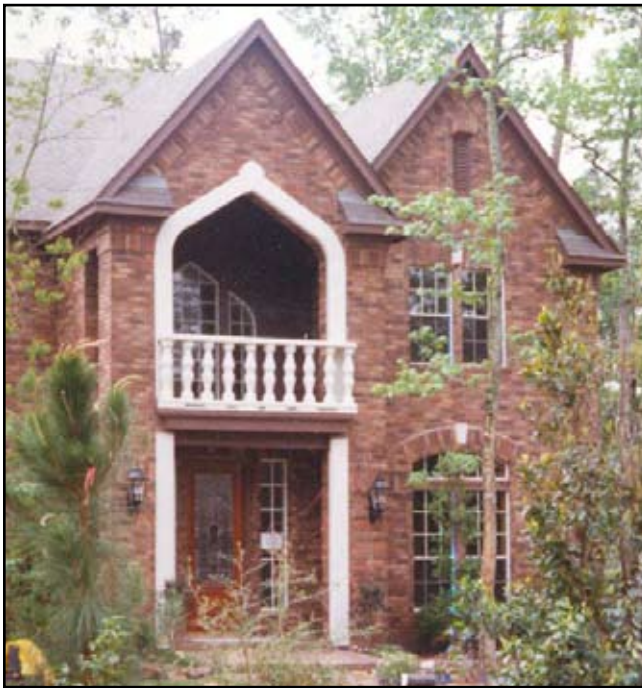
Balcony with cast arch and balustrade
