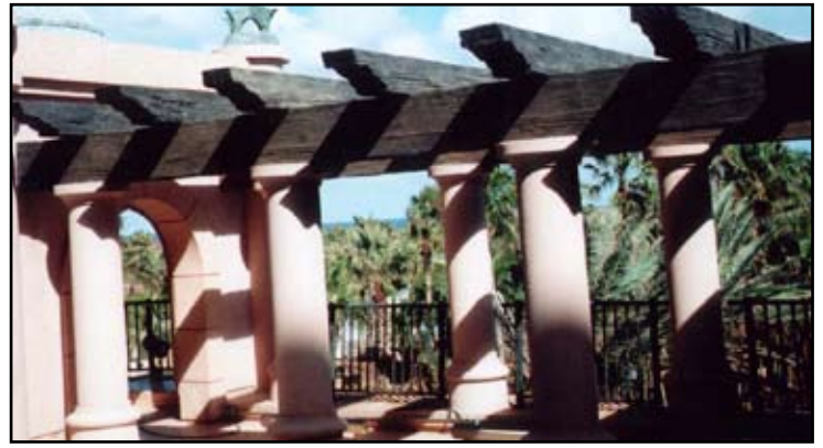
Arbor / Pergola at Atlantis Bahamas Custom columns. Beams are cast in wood timber texture in architectural fiberglass. This arbor / pergola has stood up to the tropical sun and 2 hurricanes.
